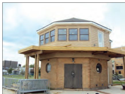
AUXTRACEN – Marcus Hook, located on the waterfront in Marcus Hook, PA, while under construction. The newly built upper floor serves as training facility, SARDET coordination, and radio watch standing.
