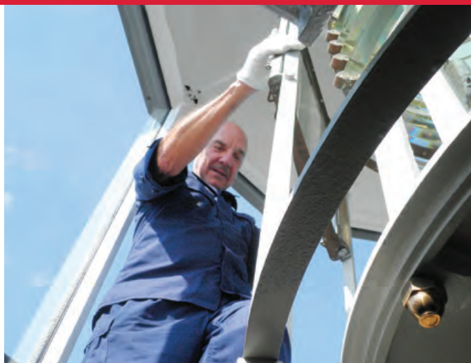
Auxiliarist Randy Irwin climbs tower to inspect and clean lighthouse.
